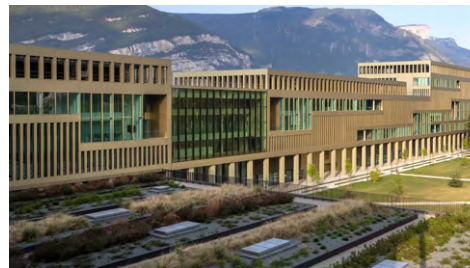
Schneider Electric, IntenCity (France)
